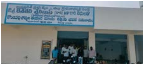
Figure 5: A newly constructed building for Kondapalli Koyu doll artisans is currently being constructed by MP Keshineni Nani Gana.
